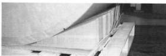
Stops can be used to secure the rolls.
